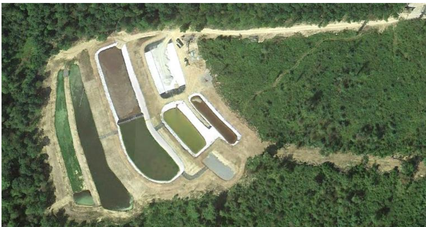
Photo 2: The Swamp Area Passive Treatment System.
