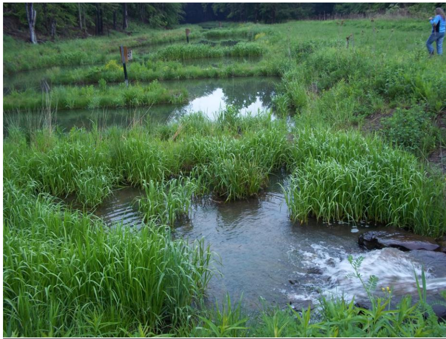
Photo 1: A constructed wetland treatment system built downstream of Stephen Foster Lake. Facilities like this contribute to the pollutant load reductions reported in Table 2 on the prior page.
